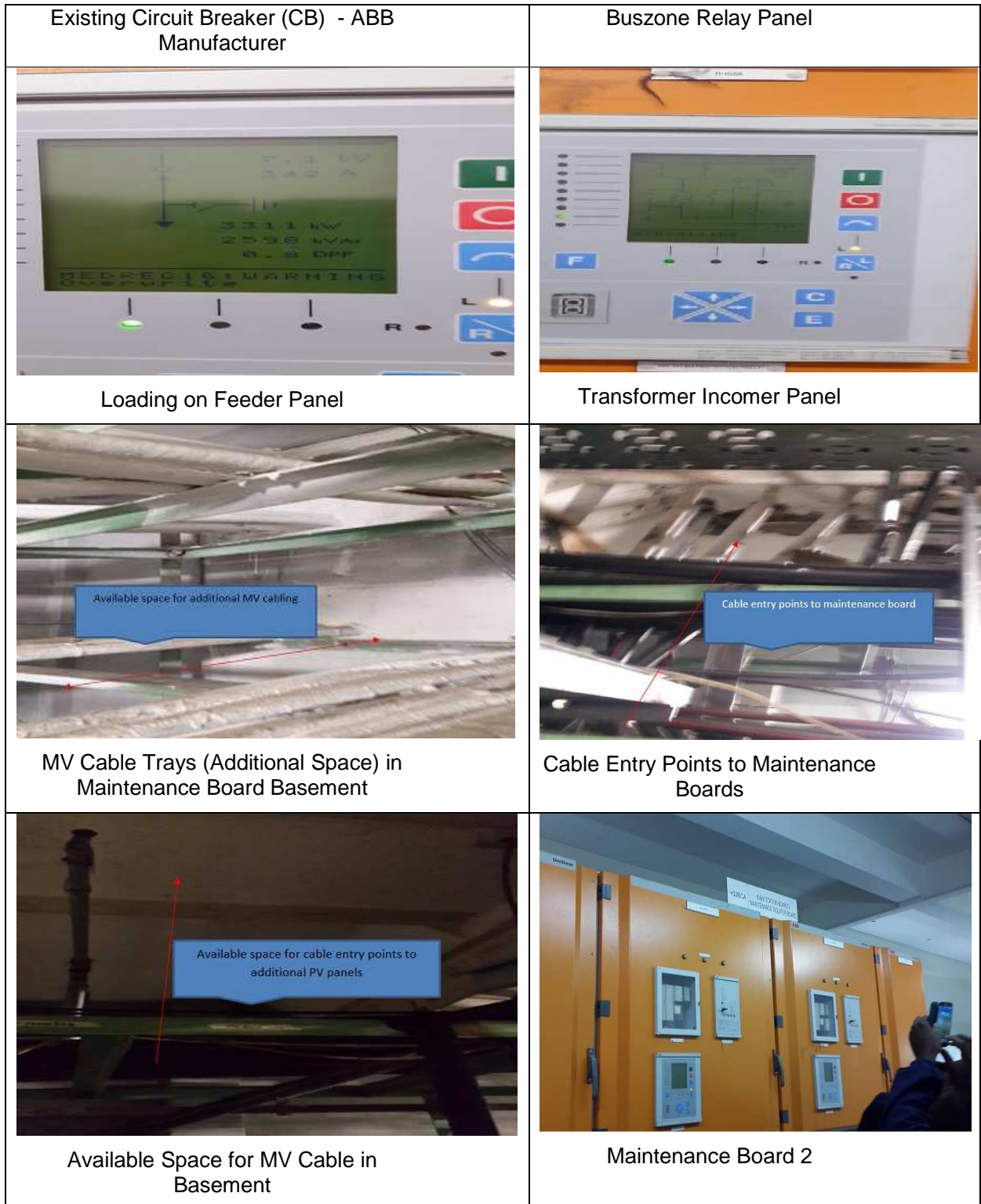
Figure 3-5: MV Cable Routing and PoC
